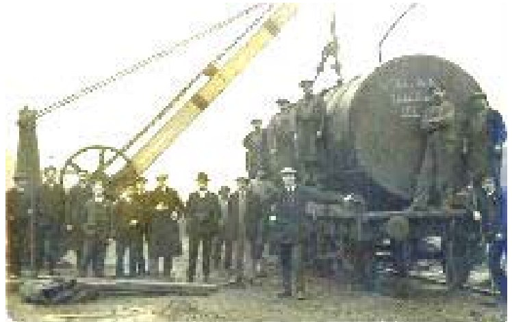
Delivery of the new boiler to the Pelabon Works through Twickenham Goods Yard, December 1914. From the personal collection of Howard Webb
